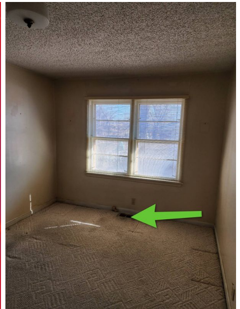
Clean All ductwork
