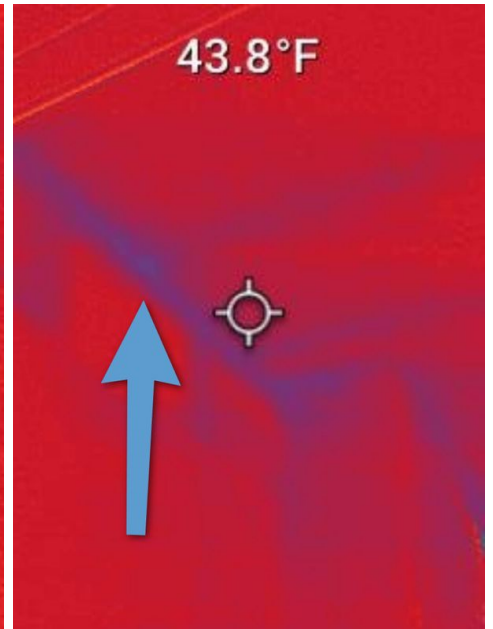
Add on hallway ceiling
